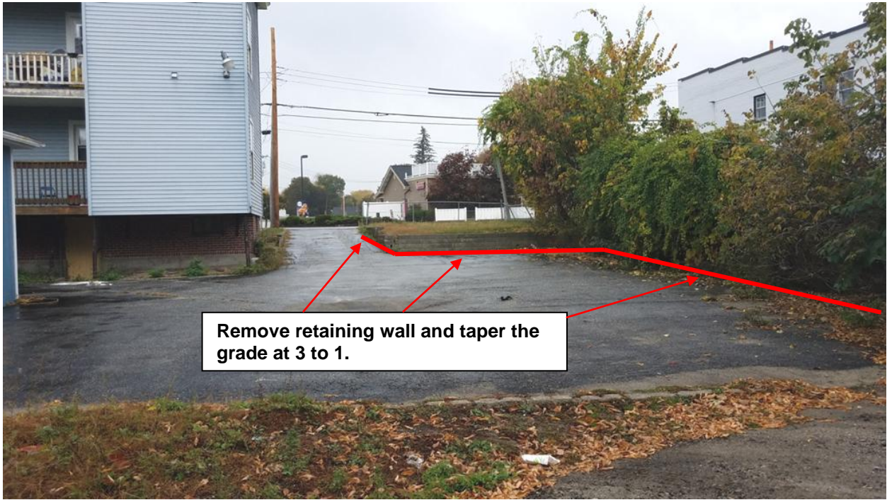
Rear View of 23 Broad St. Parking Area
